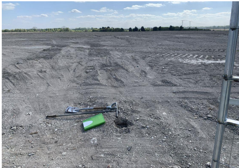
The topsoil has been spread by dozer and compacted by tracking-down.
